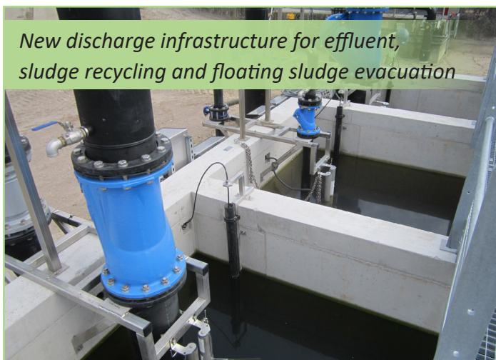
Construction of feed pipe to clarifier
