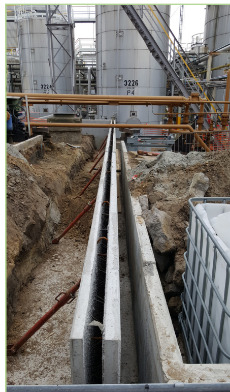
Prefab retaining wall
