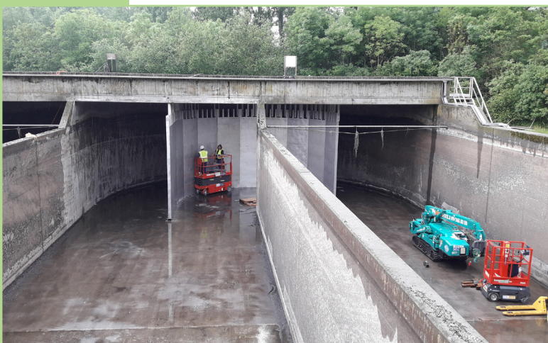
Construction of a segmented stainless steel wall
